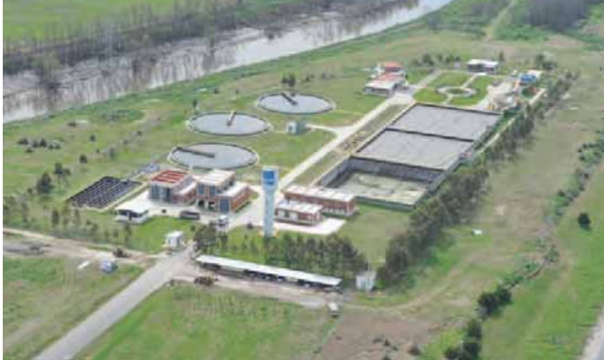
Planta depuradora Hurlingham
